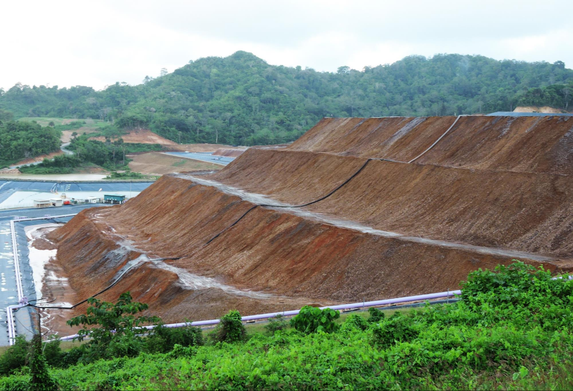
Stacked heaps 10m lifts
