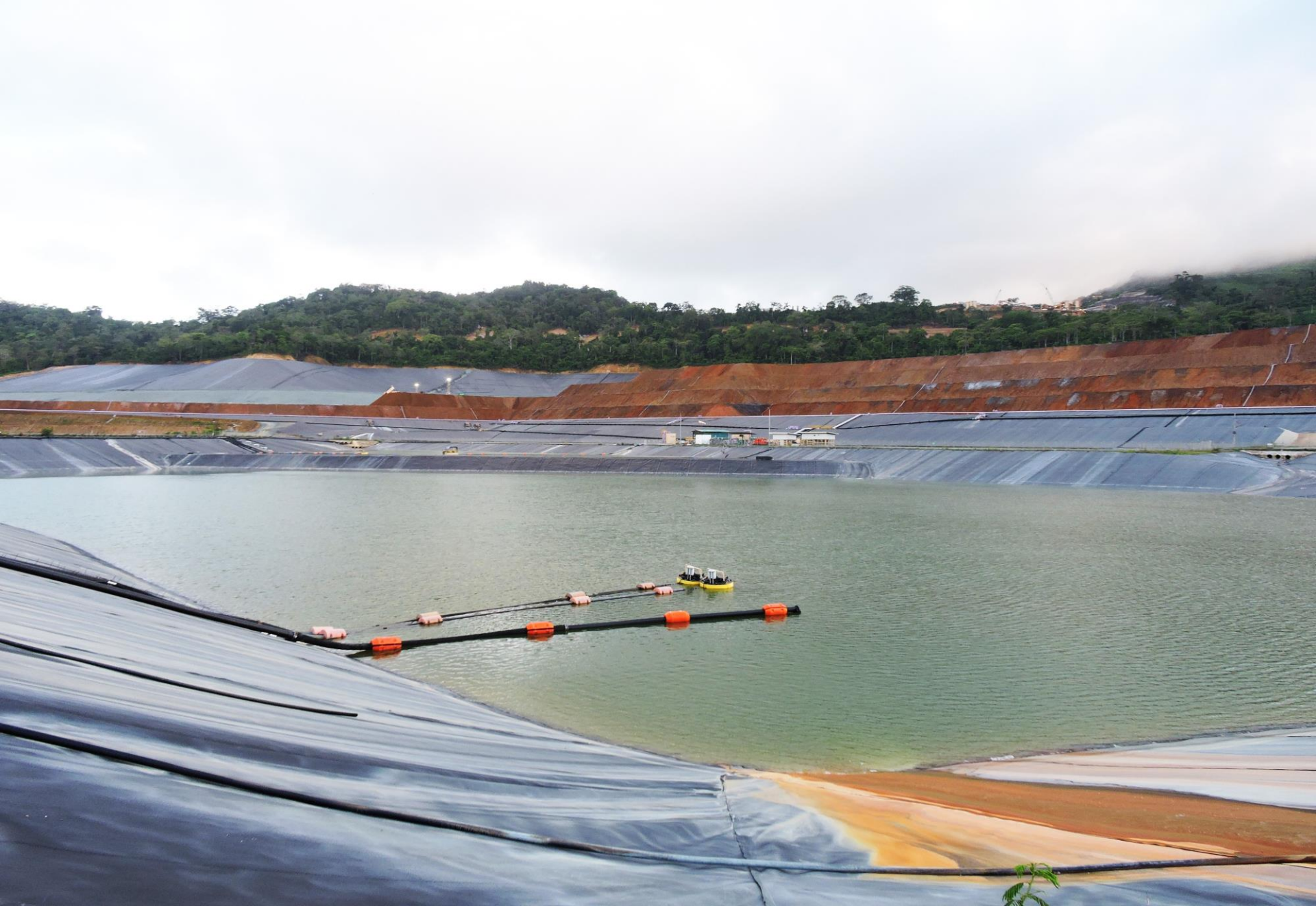
Water retention reservoir
