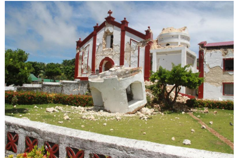
Nuestra Señora del Rosario Parish Church's damage was first reported after the M5.4 earthquake event. The church's bellfry titled after the M5.9 earthquake event (left) and finally collapsed during the M5.8 event (center, right).
