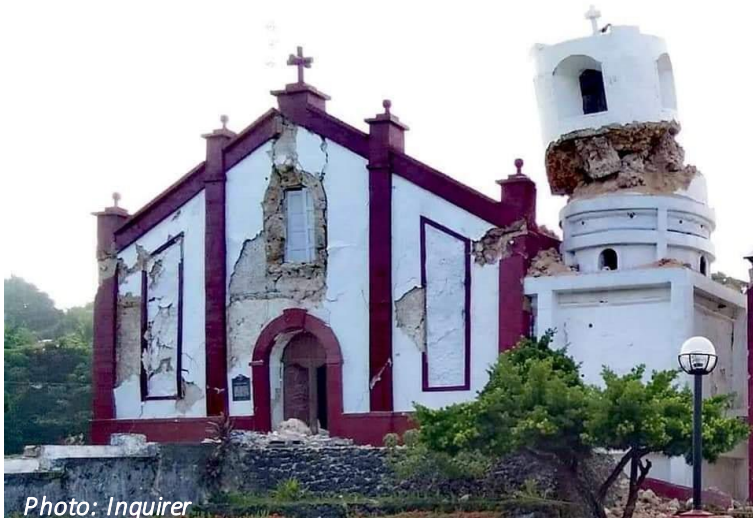
Nuestra Señora del Rosario Parish Church's damage was first reported after the M5.4 earthquake event. The church's bellfry titled after the M5.9 earthquake event (left) and finally collapsed during the M5.8 event (center, right).
