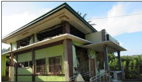
Brgy. Paraiso Birthing Hall
