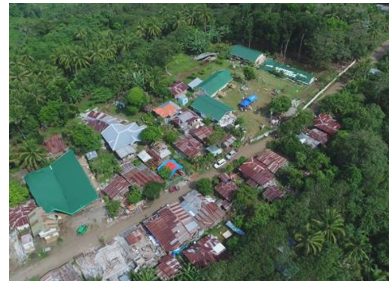
Drone photo taken by PHIVOLCS QRT at Bgy. Daig, Tulunan
