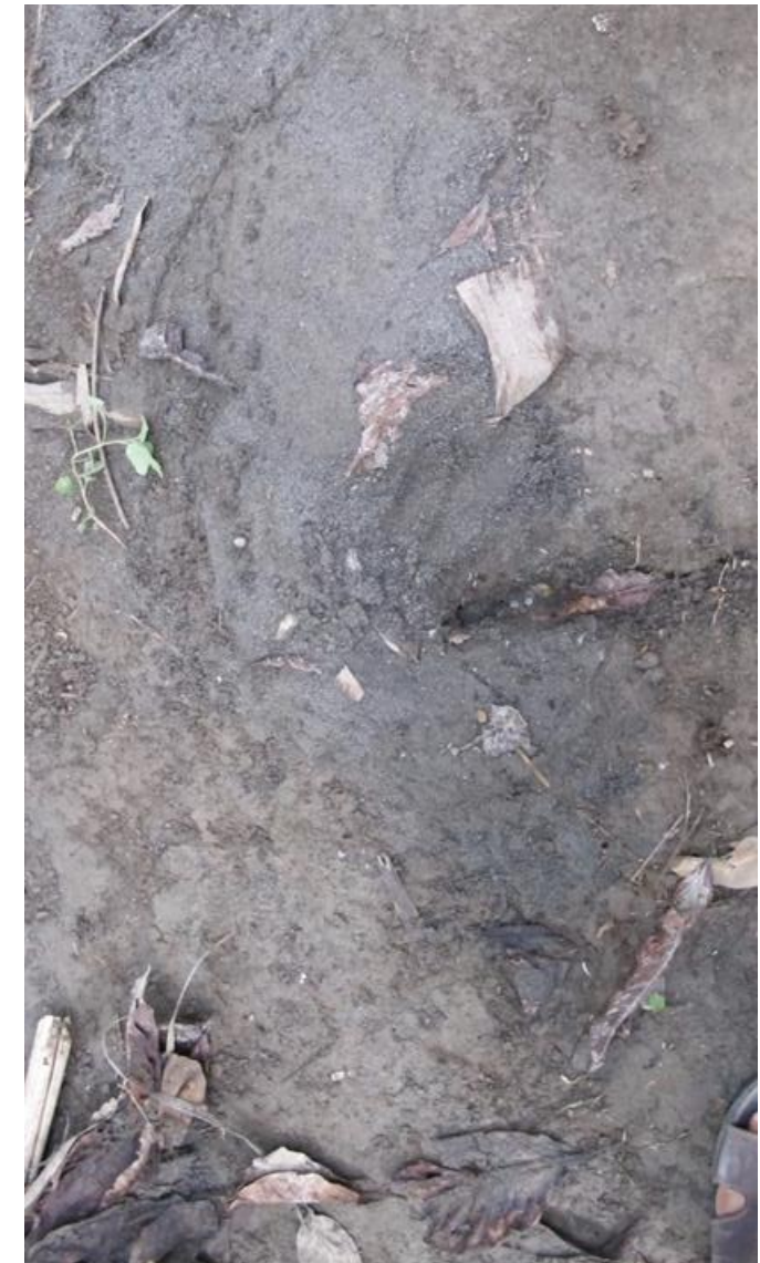
Sandboils observed in Brgy. Tamlangon after the M6.6 earthquake
