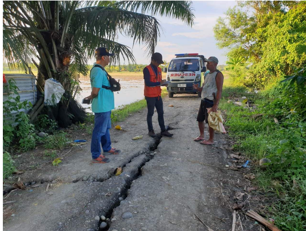
Lateral spread and sandboil
