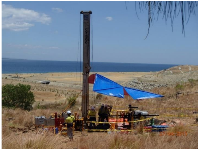
Geotechnical drill rig
